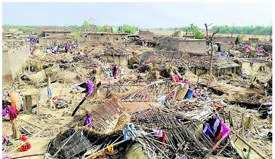
Figure 2. Destruction of homes in Purainiya village of Parsa district of Nepal caused by the storm on 31 March 2019. (Source: https://myrepublica.nagariknetwork.com/news/10-latest-developments-on-bara-parsa-tragedy-with-photos/ .)
